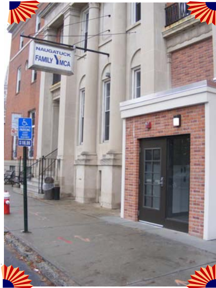
Elevator Street Entrance
